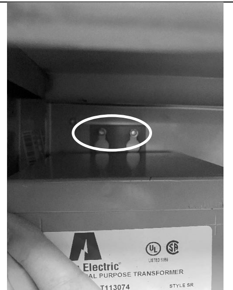
c) Tighten the mounting screws.
