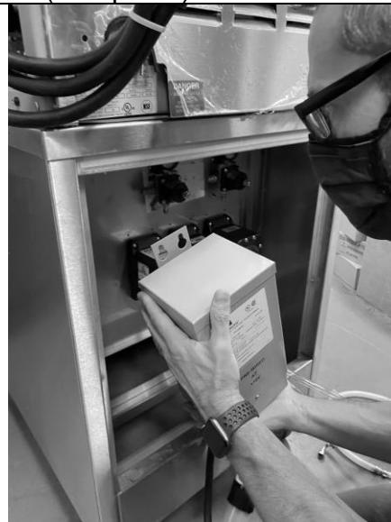
b) Carefully hang the transformer on the mounting screws.
