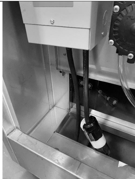
e) Connect Viper power cord to transformer.
